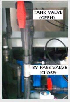
8. Fix the flowing rate and the R/O pump pressure for the right operating condition by turning the FLOW CONTROL VALVE to the right side slowly
