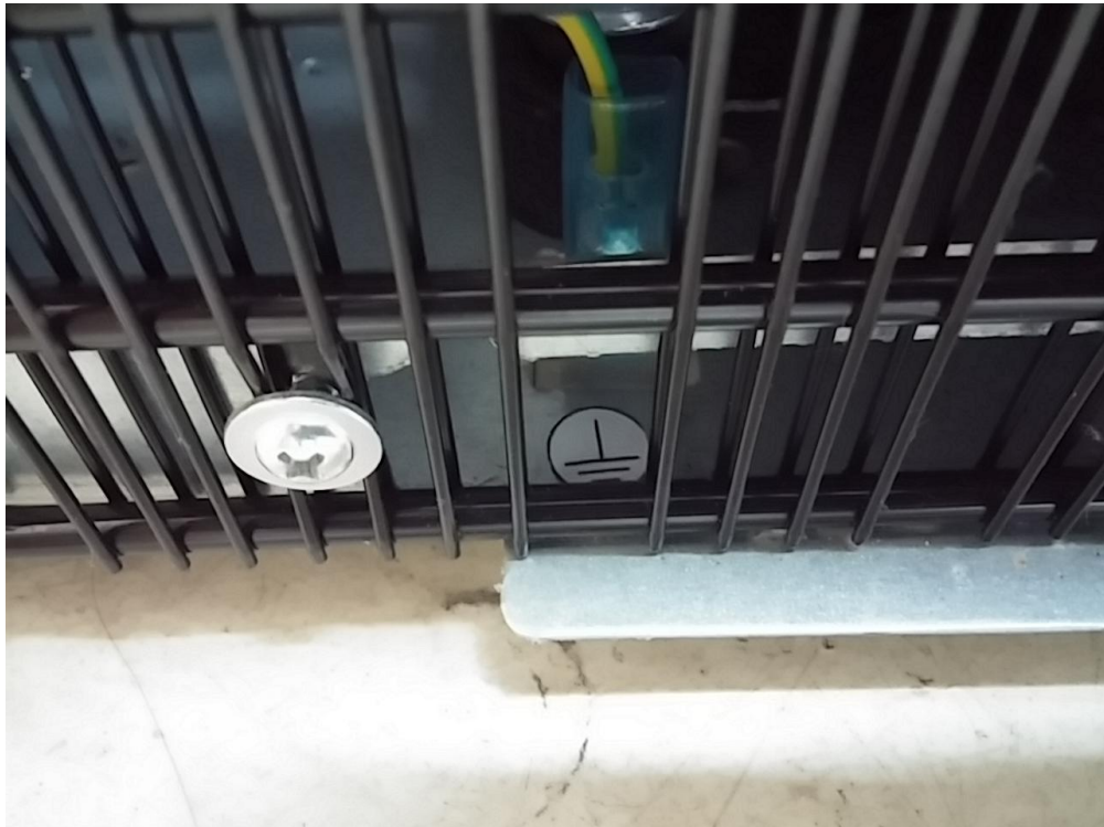
<Protective earth connection>
